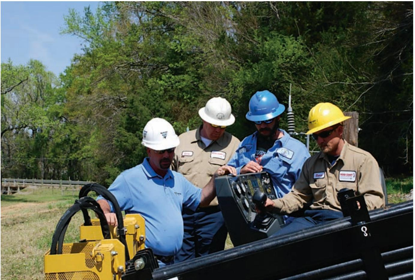
**Chance Holland, seated, operated the boring machine, which is used during underground electrical construction, while others looked on.**
