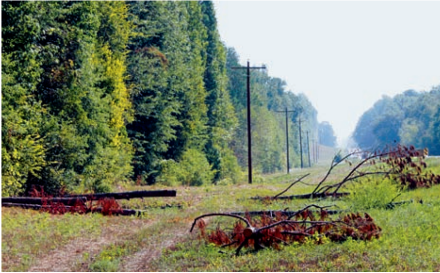
Downed trees near power lines illustrate the importance of a vigilant right-of-way program. A well-maintained clearance greatly reduces interference with the delivery of electricity.
