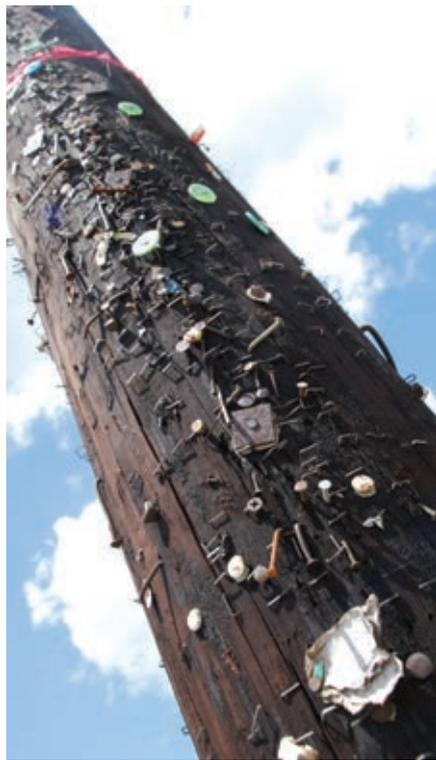
**This beleaguered WCEC power pole has been plastered with countless unauthorized attachments, resulting in a dangerous condition caused by sharp staples, tacks and nails.**
